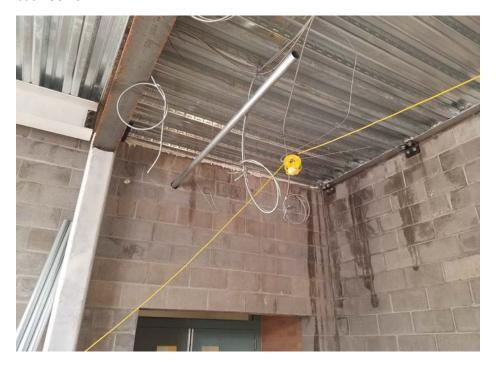
Tension rods have been installed to support the roof of the structure. There is a little more roof work that needs to be done and then the exterior portion of this project will be done.
