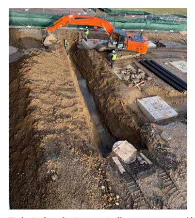
The footing forms for the new main office area were prepared for the pouring of concrete.
