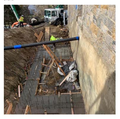
The framing of the new wing was started. Surveyors staked out the footings for the new structure.
